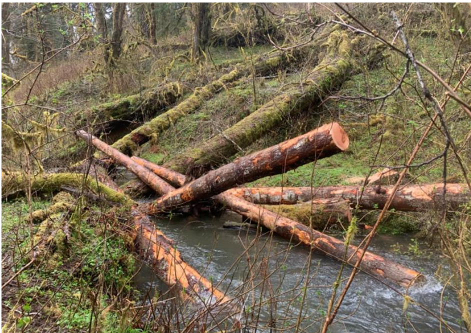
Large woody debris placement, Nehalem River watershed (ODFW)
