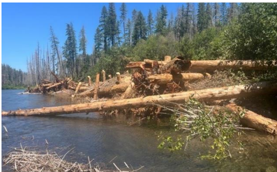
Large wood jams were installed to reshape the river channel and bring year-round water flow back into a historic side channel.
