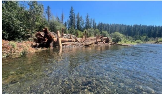
Large wood jams were installed to reshape the river channel and bring year-round water flow back into a historic side channel (continued from previous photo)
