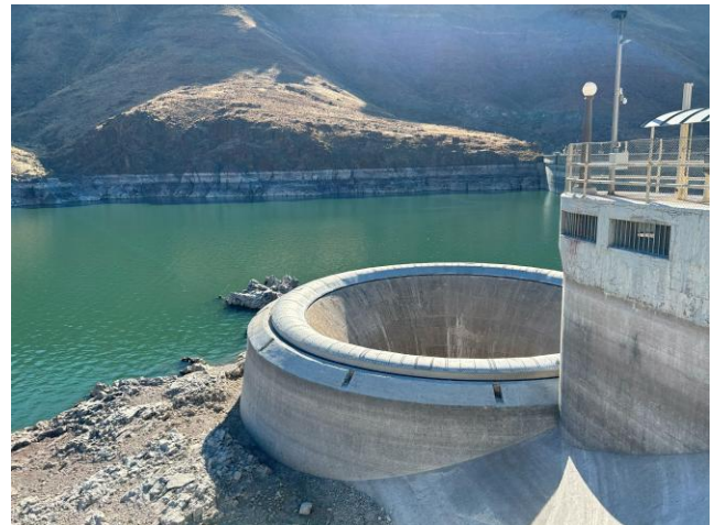
Lake Owyhee Dam's Morning Glory spill hole as seen with low water during Sept. 2025.
