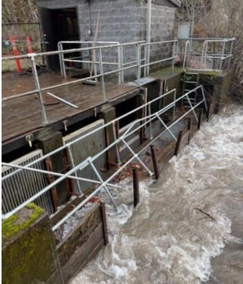
The bent railing is usually where staff stand to clean the screens at Cascade Hatchery. The wooden deck above was submerged at the highest river level.
