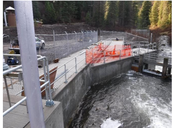
View of Lookingglass Creek flowing downstream through the newly constructed fish ladder at the hatchery.
