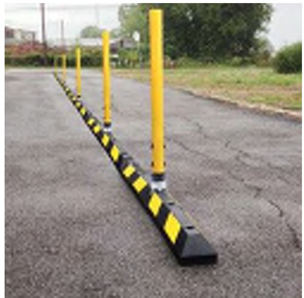
Figure 10 - Rubber Delineators (Source: sealcoating.com)
