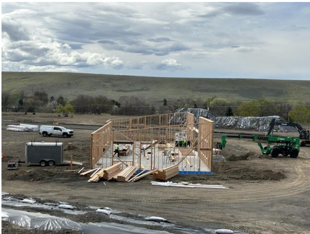
Status of office construction as of April 2, 2026.
