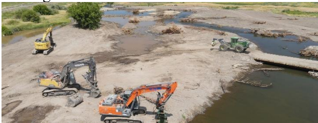
Ochoco Preserve project construction, 2024. Photo by DLT.
