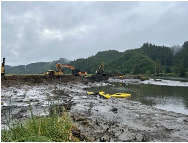
Excavators break through the levee, restoring a wetland after 130+ years.
