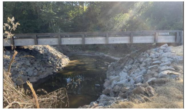
A new bridge replaced the old culvert, allowing all native fish species to move freely in Pheasant Creek. Photo credit: John Hanson, ODF.
