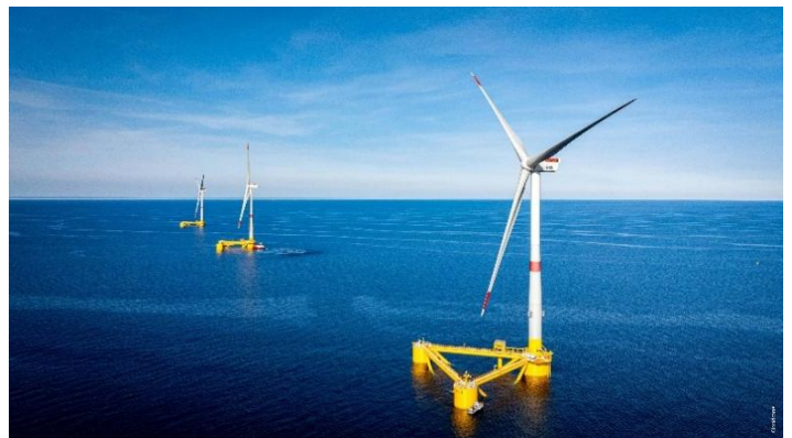
These 10 MW floating turbines are the largest in the world and are similar to what may be proposed in the future off Oregon. The 30 MW Éoliennes Flottantes du Golfe du Lion (EFGL) project is in the French Mediterranean operated by Ocean Winds. Image courtesy of LEFGL/Ocean Winds.
