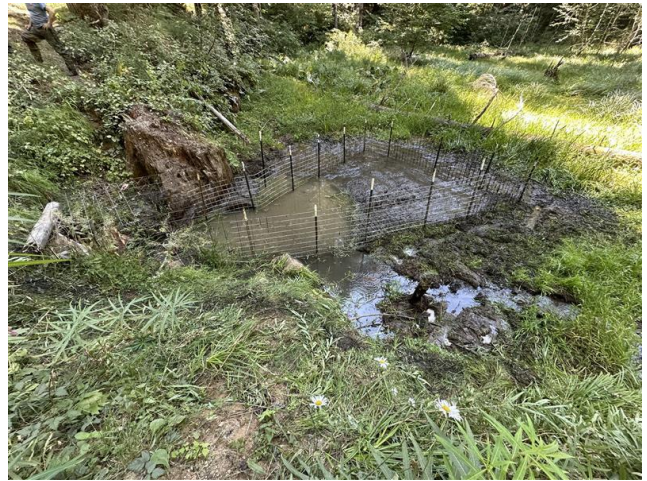
The new device ensures water flow while excluding beavers.
