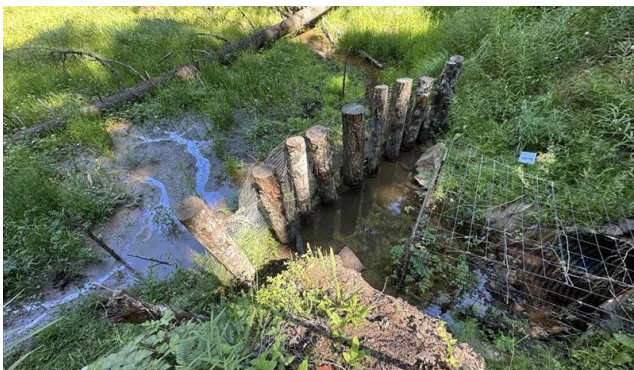
This photo shows the old culvert protection device before replacement.
