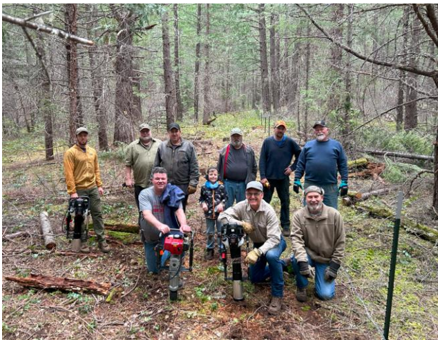
OHA members from five different chapters volunteered their time to replace dilapidated fencing in the Southwest Cascades.
